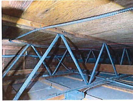
FYI - Attic space
