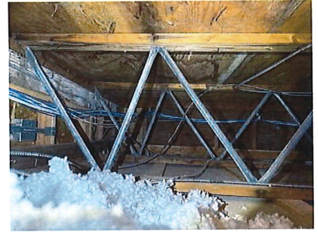
FYI - Attic space
