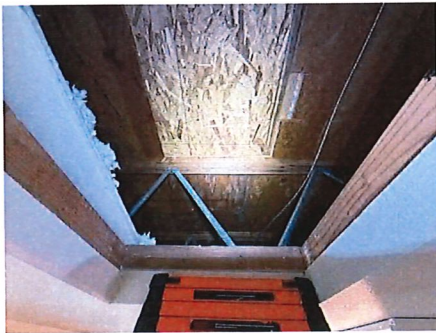
FYI - Attic space
