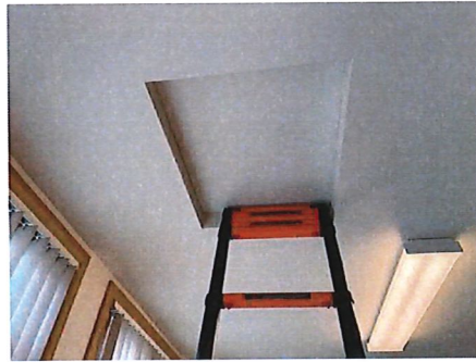
FYI - Attic space access in conference / break room
