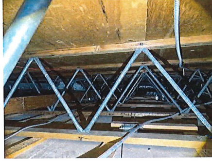
FYI - Attic space
