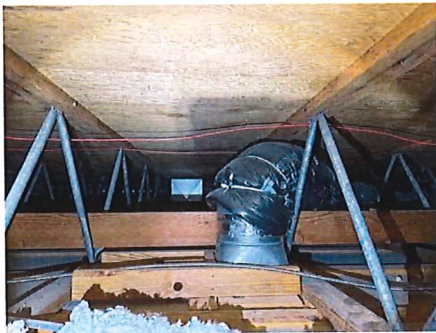
FYI - Attic space
